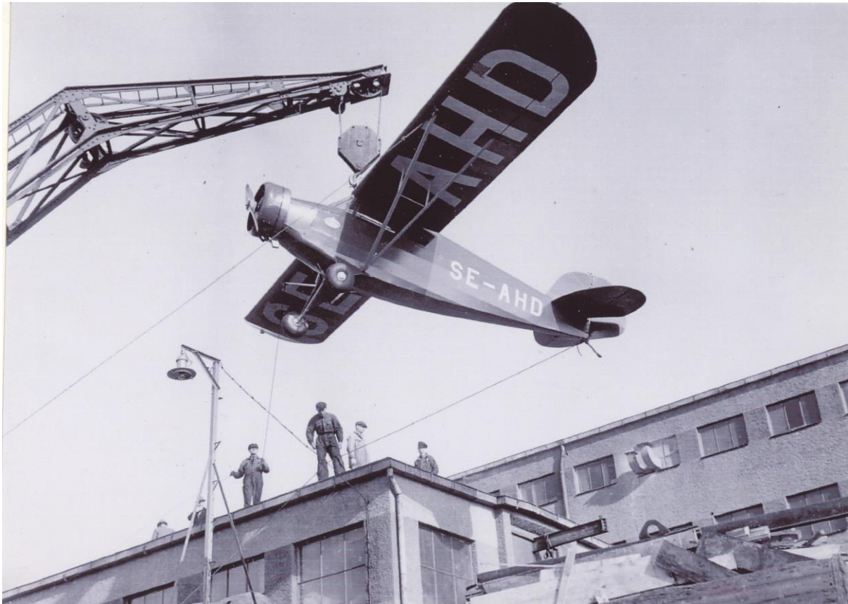
The second production GV-38, SE-AHD, being removed from the assembly hall. Photo: via Per Björkner
